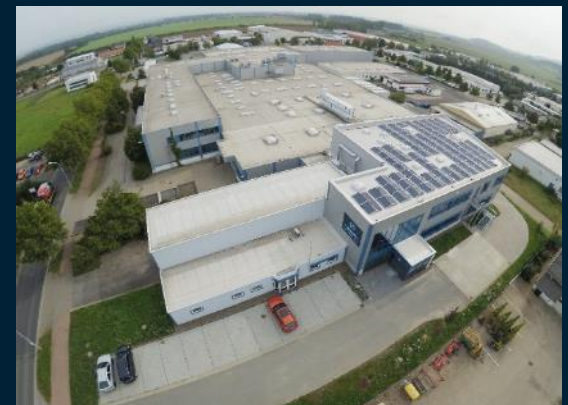
Production facility in Wernigerode
