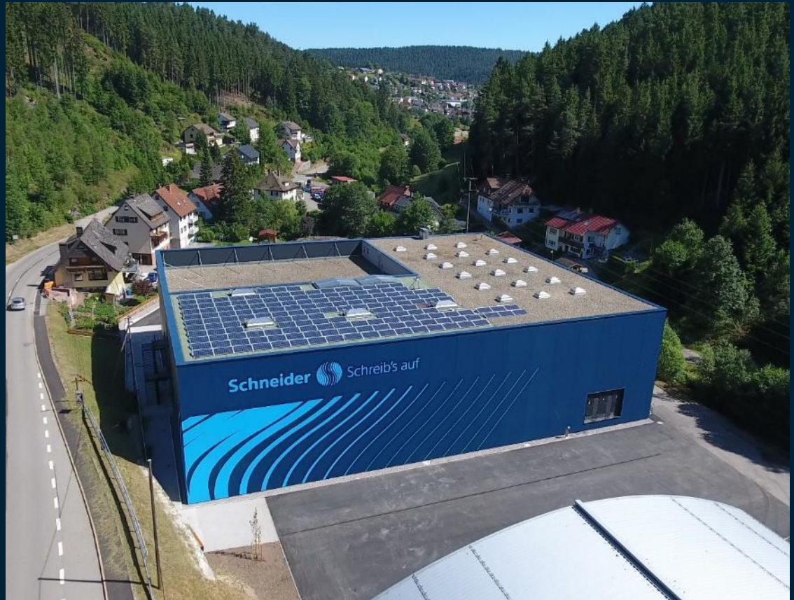
Photovoltaic installation on the roof of the warehouse/logistics building blulog
