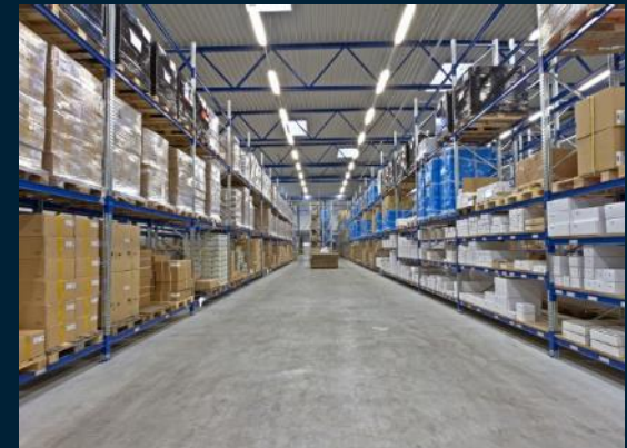
Waste heat for heating warehouses
