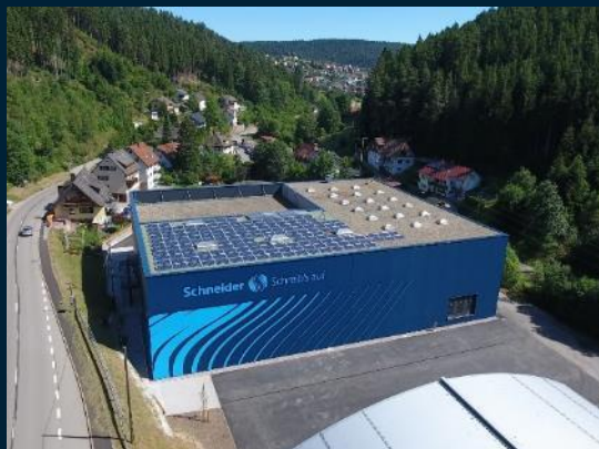
Logistics facility blulog in Tennenbronn
